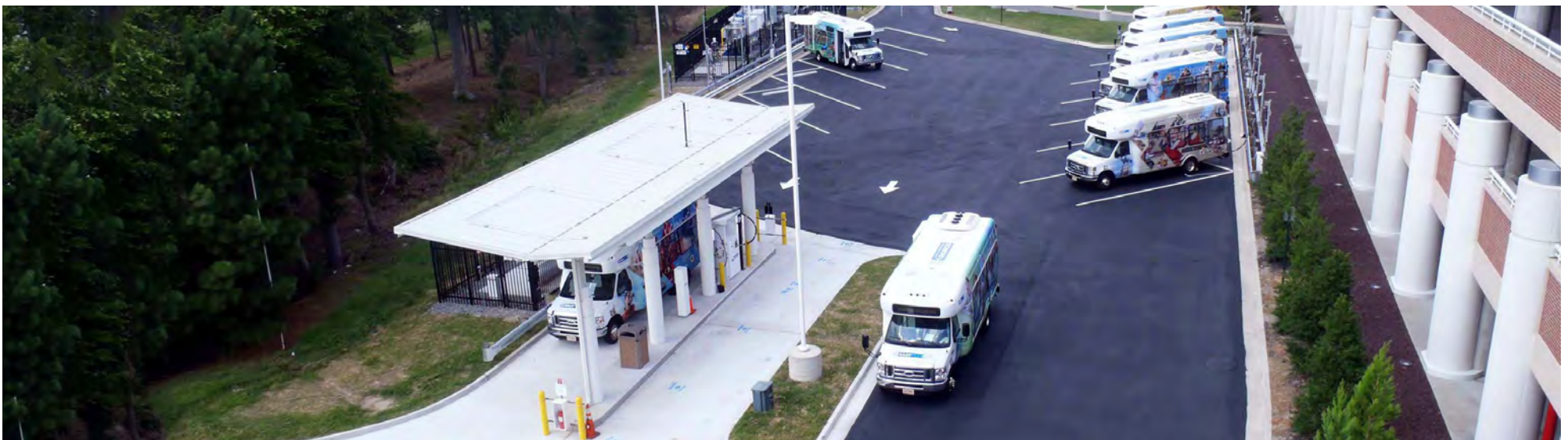
CNG refueling station, Richmond International Airport
